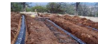
Layout pipelines and marking inverted levels (P4)
